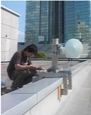
Aleph Networks Technician Installing Gigalink Interop Tokyo, 2009
